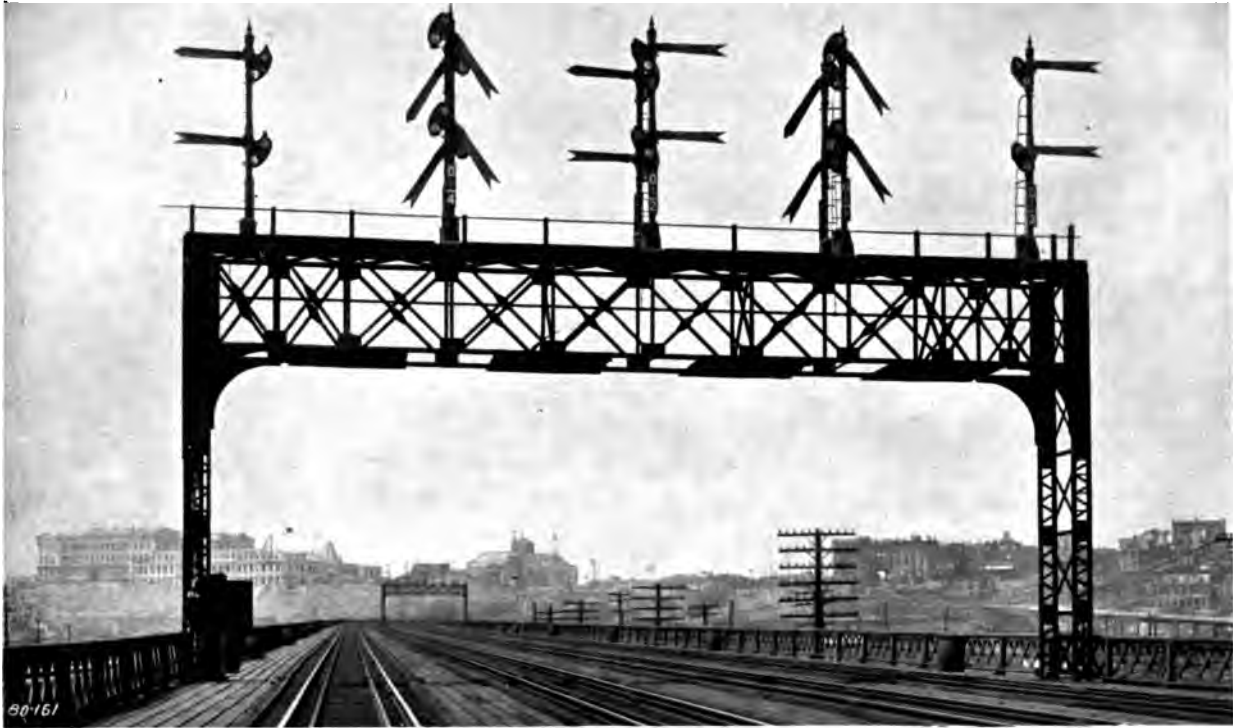
Signal Bridge on Viaduct East of Bergen Archways, Erie Railroad.
